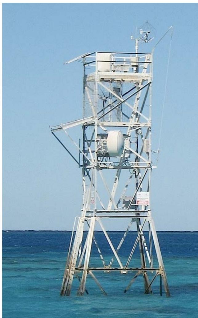
Figure 2. The weather station at Davies Reef. The microwave dish is in the centre of the image. The solar panels for the power system are on the left, the wind turbine is in a bird proof cage on the third floor. Enclosures housing system electronics are obscured by the microwave dish.
